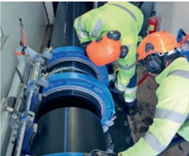
Minimal ovality is a condition for safe joints and efficient operation.
